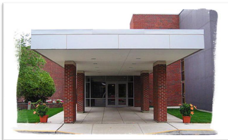
A canopied entrance with drop off area and curb cut allows safe and easy access at 2006 TEAM W Award winning Temple Jeremiah, Northfield, IL.
